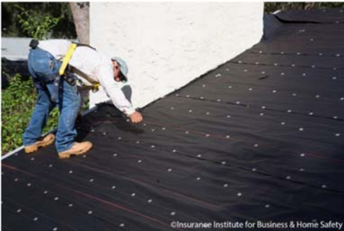
Sample Photo 3: Underlayment Nailing
