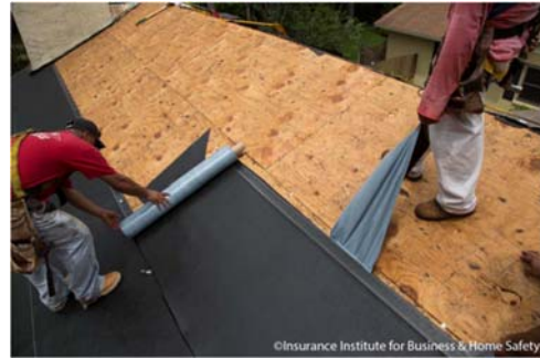
Sample Photo 4: Underlayment "peel-and-stick"
