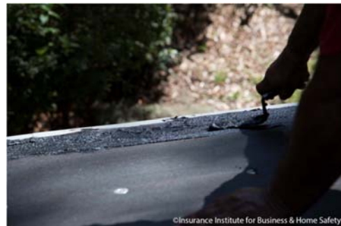
Sample Photo 5: Mastic Application Over Drip Edge for Starter Strip Adhesion
